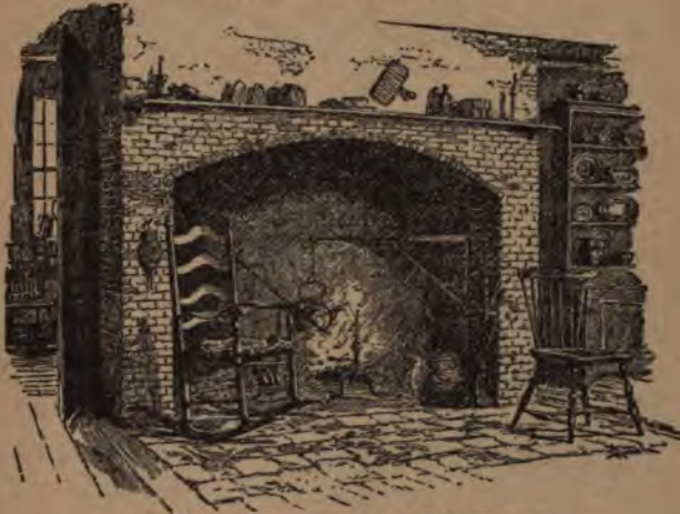
General Washington's Fire Place.
